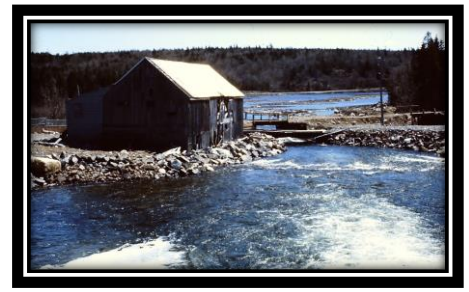
1970's - The last Days of the Pockwock Mills. The Haverstock Brothers Mill on Pockwock just before it was demolished - 1974
